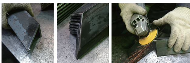
before grinding after grinding grinding
