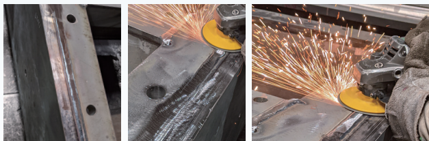
before grinding after grinding grinding
